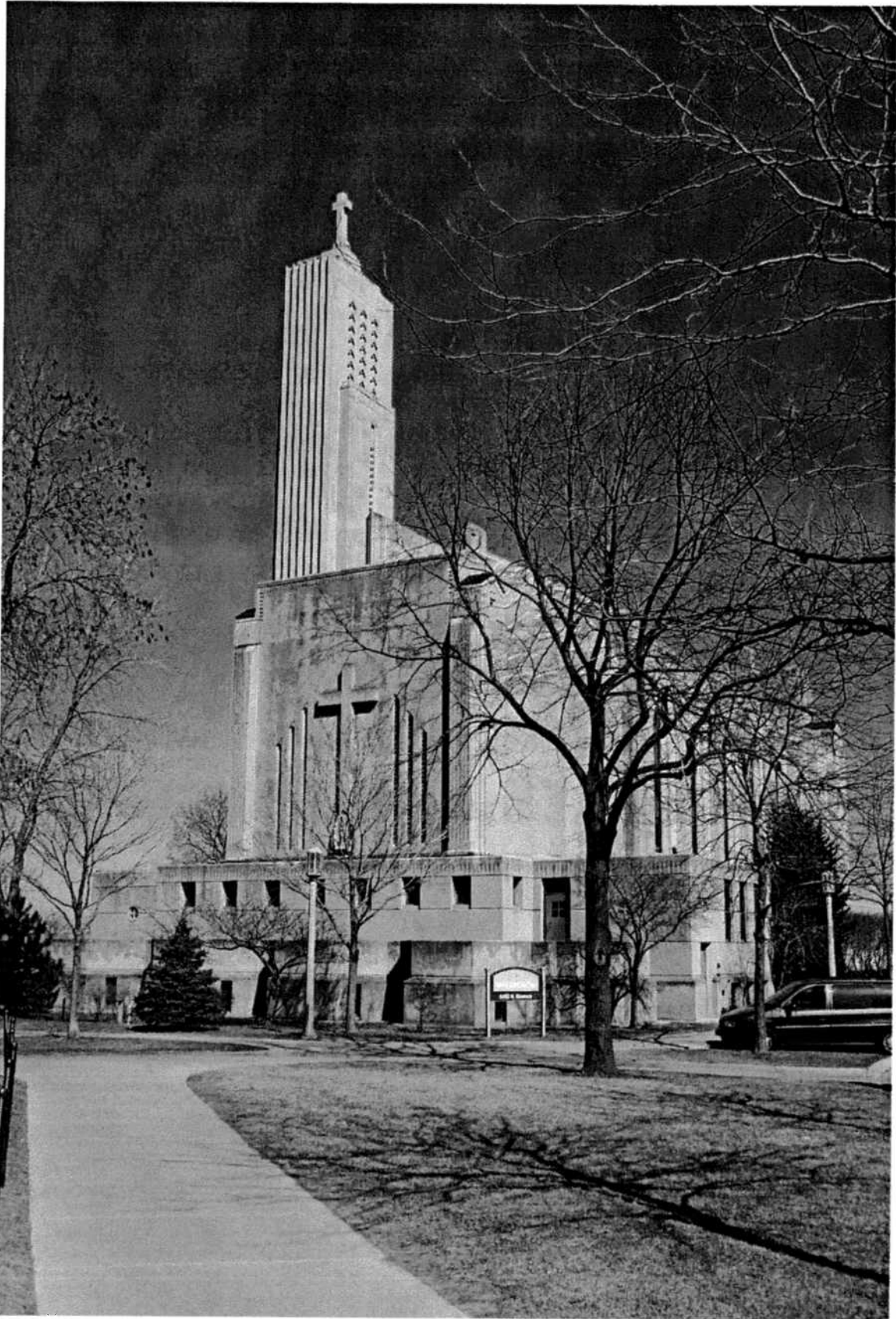
A view of Madonna della Strada Chapel (rear elevation) from the southwest.
